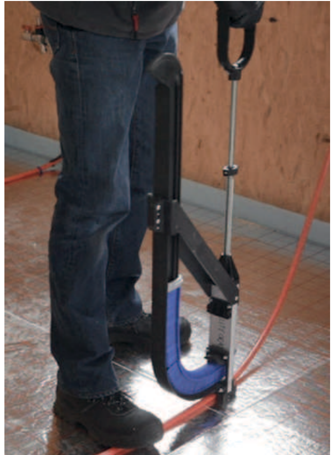
installation with staple system
