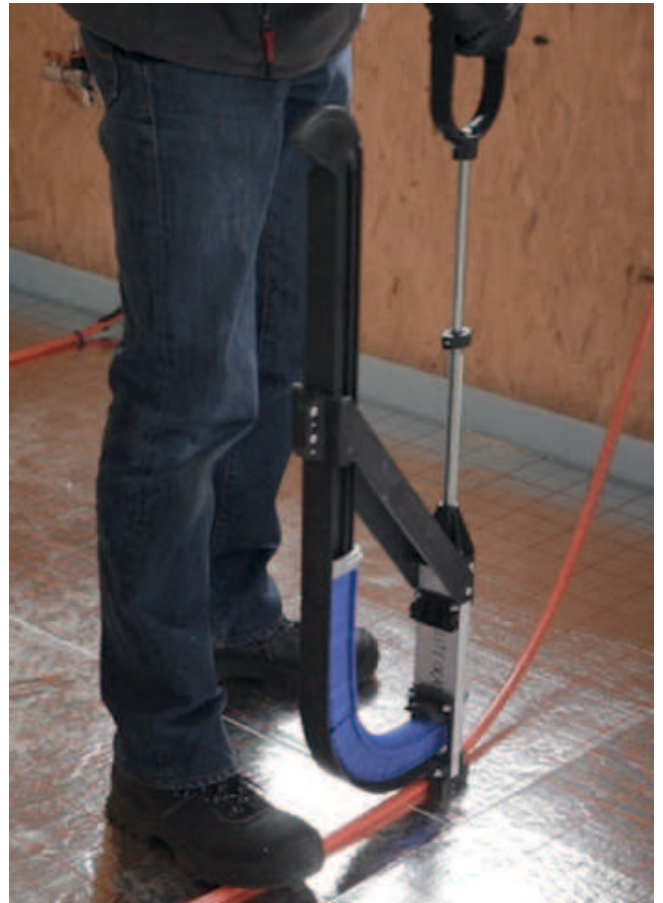
installation with staple system
