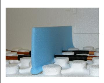
punch holes in the PE expansion joint plate for snap-in panels NPPED with self-adhesive tape (130 mm = 5 1/8" high, 10 mm = 6/16" thick, foot 24 mm = 15/16" thick) where pipe runs and then push it into the snap-in panel
